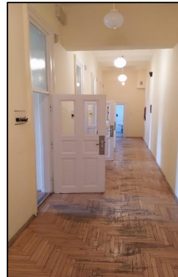
Corridor with worn floorboards
